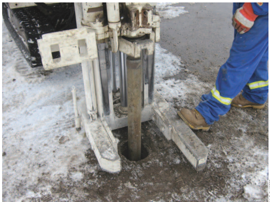
Foreuse type, Phase II
